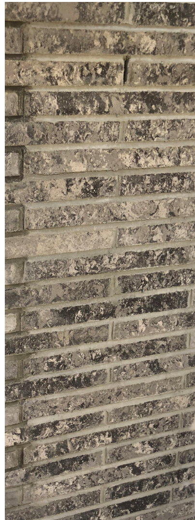
3. Mottled grey masonry brick stacker bond
